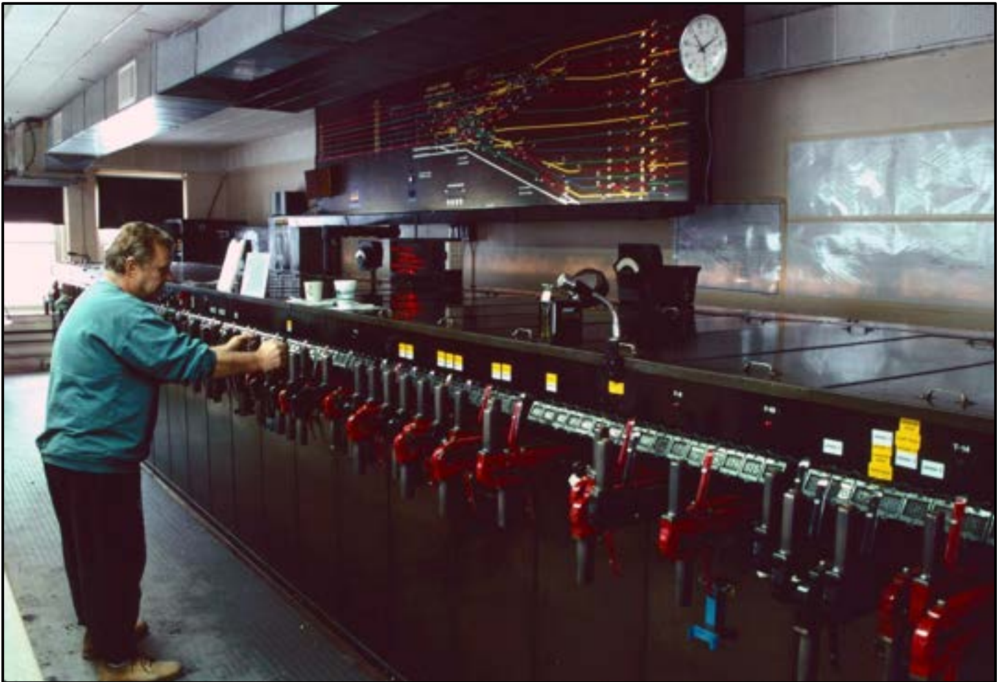
Rows of levers – red for signals and black for switches – line the outside of a control box at the John Street facility (Steve Bradley photo)
